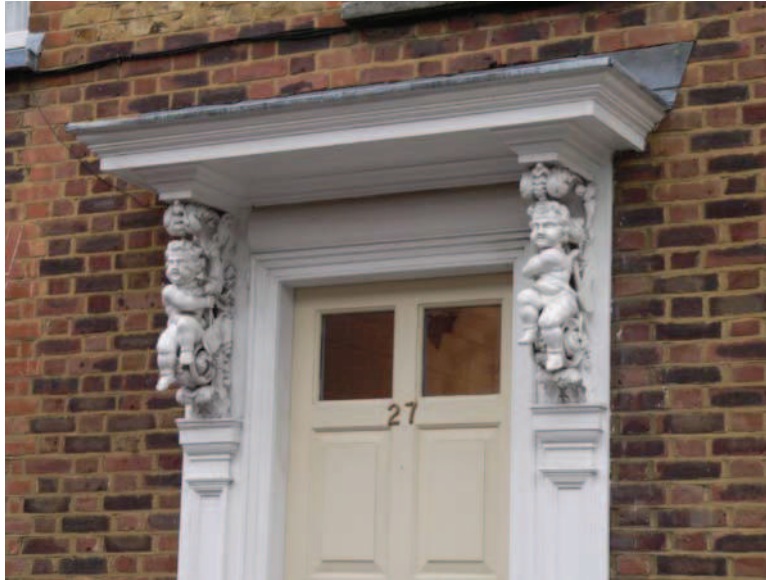
Architectural detailing, Deptford conservation area
